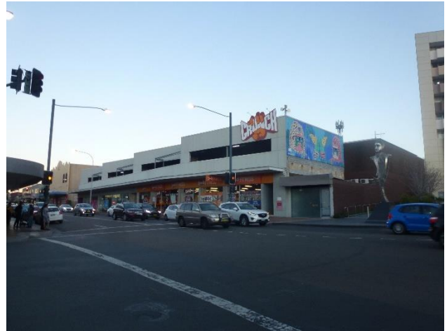
Figure 5: Commercial building occupying the site as viewed from Scott Street (north west)
