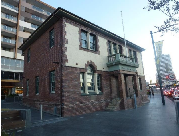
Figure 19: Memorial Arts Building
