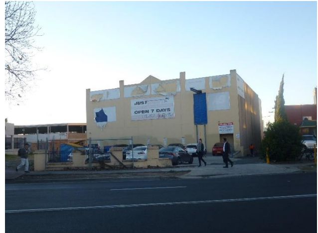
Figure 10: Existing development from the south east
